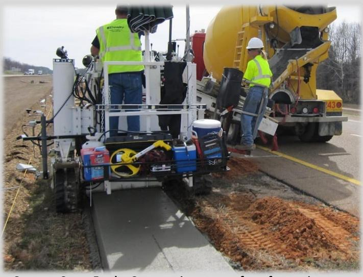
Concrete Screw Feeder Conveyor increases safety of operating crew.
