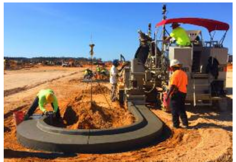
Pouring curb & gutter with 3-D (stringless) control.
