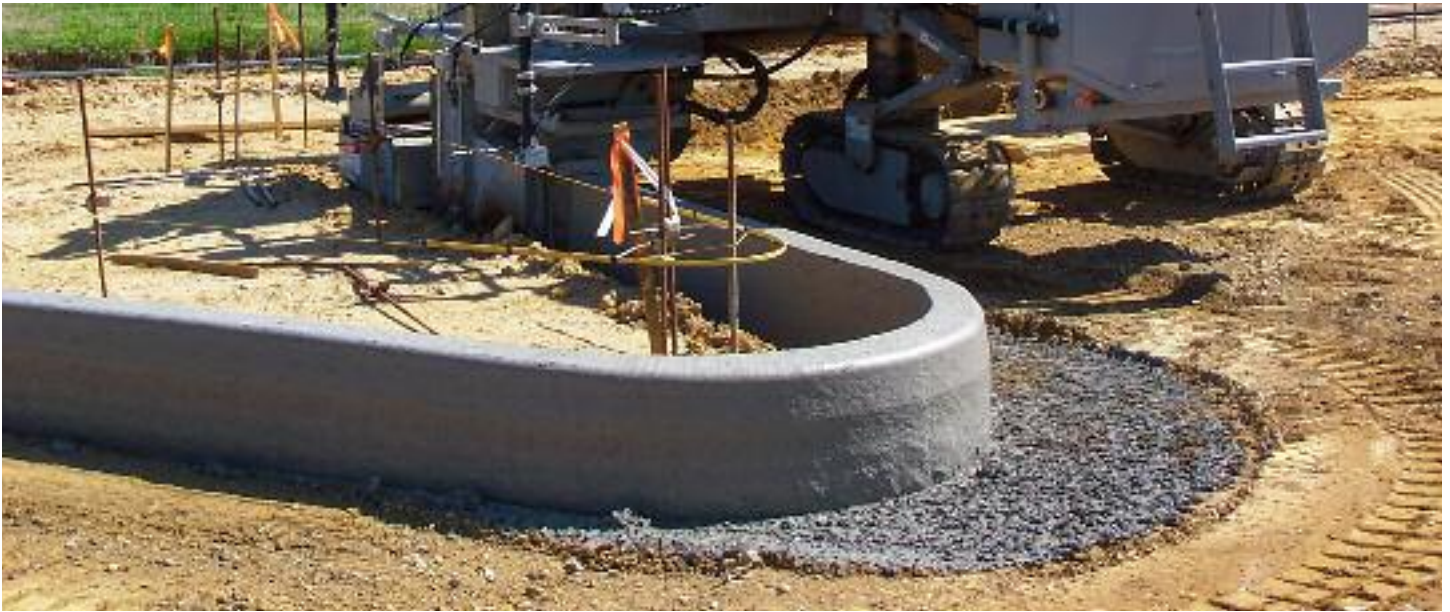
The machine's tight radius capability eliminates hours of hand forming and produces a higher quality product.
