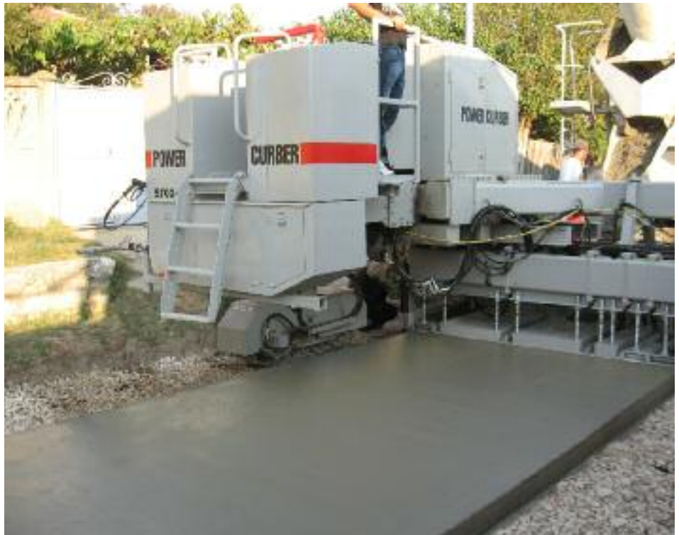
Paving 10' (3m) wide. Center pour paver is sectional for varying paving widths.
