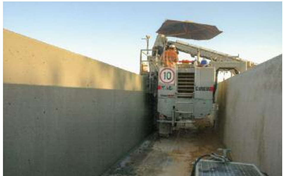
Canal in Australia, base 12' 5.5" (3.8m) wide and sides 6'10" (2.1m) high. (Shown with custom belt conveyor)
