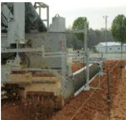
Custom trencher trimmer and poultry house foundation.
