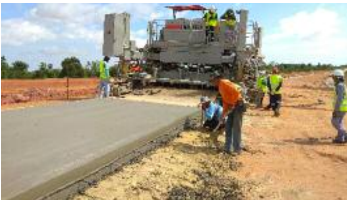
▲ Power Curbers 7700 Multipurpose Slipform Machine Paving
