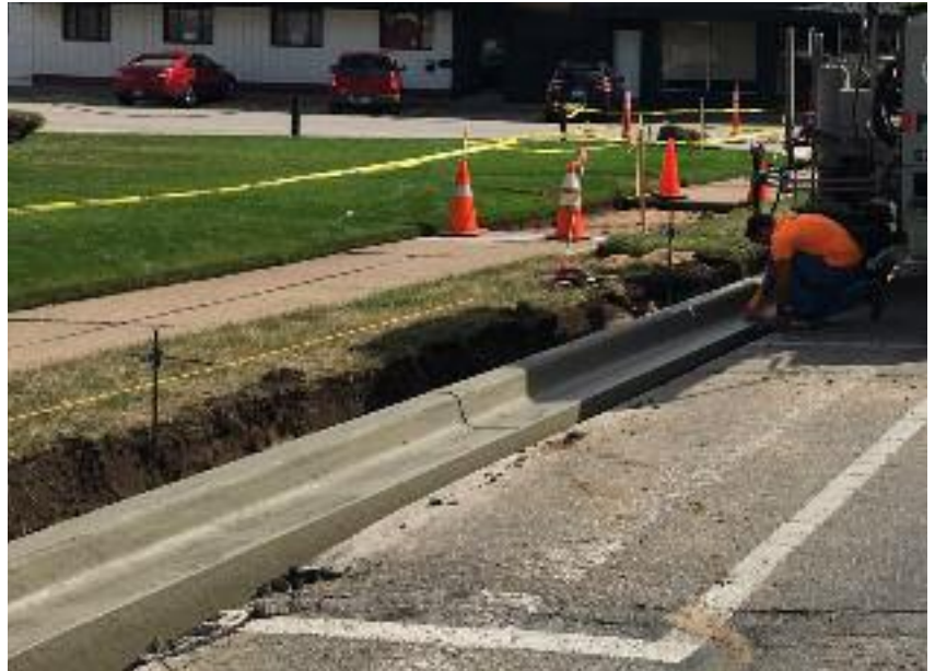
Curb & Gutter in a rehab application
