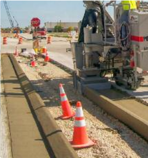
Tapered curb & gutter, poured over dowels adjacent to the pavement.
