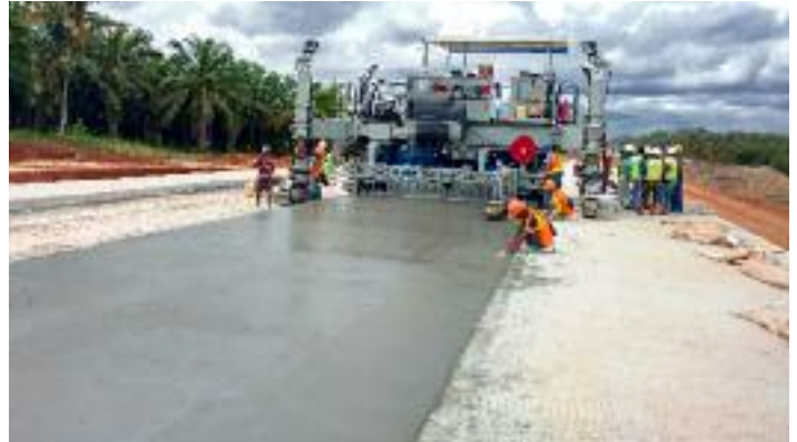
▲ Power Pavers Full-Sized, 4-Track SF-2404 Slipform Paver
