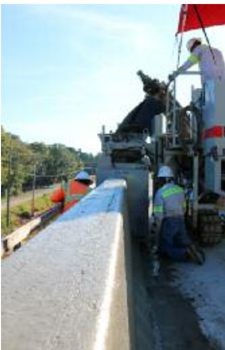
Close up of Bridge Parapet
