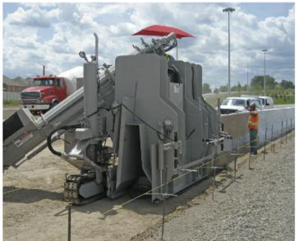
MAX package pouring large variable barrier wall.
