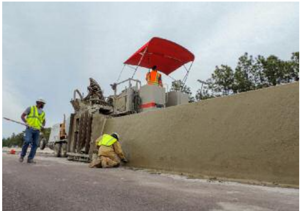
Variable barrier, up to 58" (1.47m) tall.
