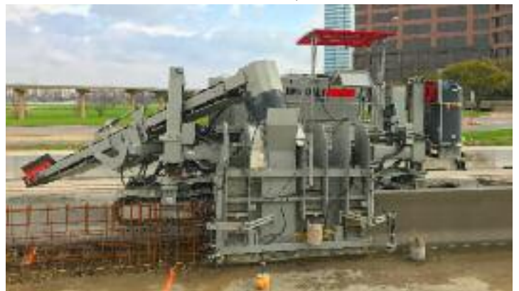
▲ Power Curbers 7700 Multipurpose Slipform Machine Pouring Variable Barrier
