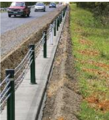
The 5700-D is an all-in-one solution for installing no-mow strips for cable barriers.
