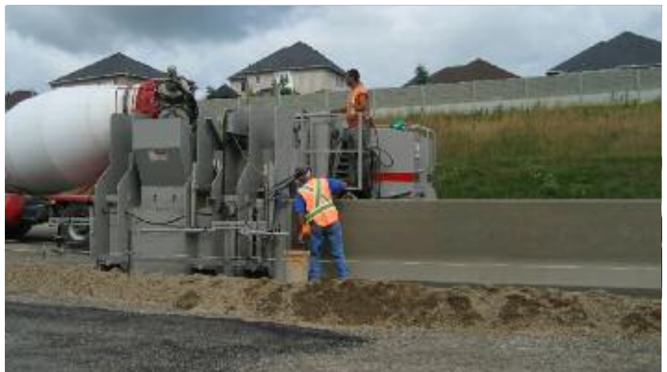
Variable barrier, up to 68" (1.72m) tall.
