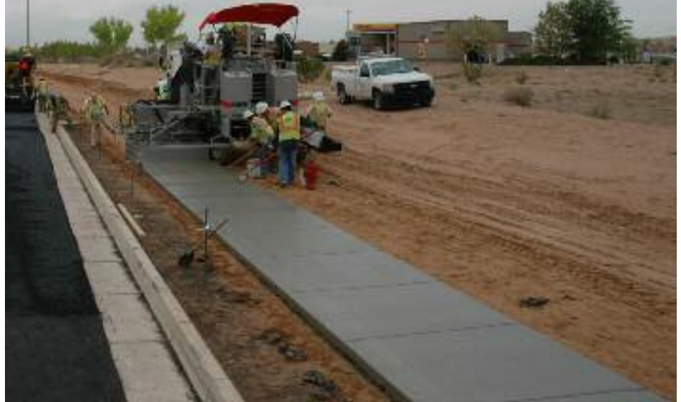
Pouring a 6' sidewalk.
