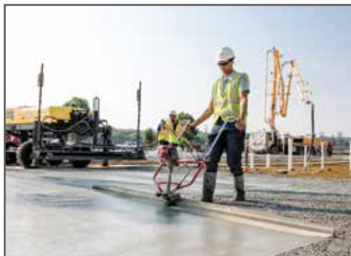
The unique, patented blade simultaneously cuts and smooths concrete.
