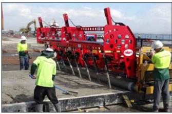
For over twenty five years, Allen has been the preferred source for triple roller tube pavers. These unique form riding machines can do the work of larger more expensive pavers in many applications. Triple roller tube pavers are easy to transport and setup as they have lighter weights than traditional slip-form pavers. These pavers are great for confined, urban job sites where forms are going to be used or concrete streets, parking lots, shoulders, ramps, approaches, airfields and more.
