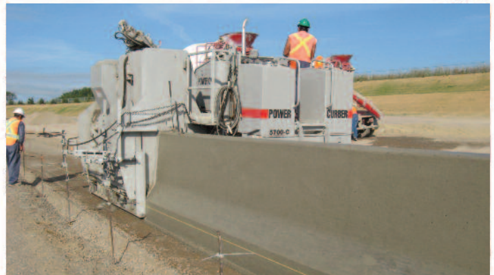
▲ Power Curbers 5700-C Slip-Form Curb Machine
