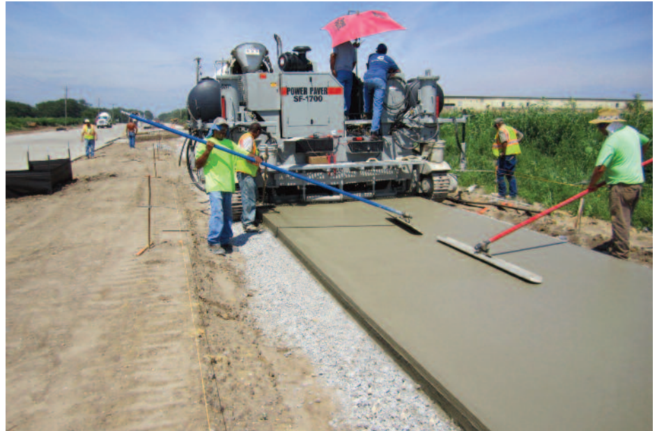
The minimum paving width for the SF-1700 is 9 feet or 2.75 meters.
