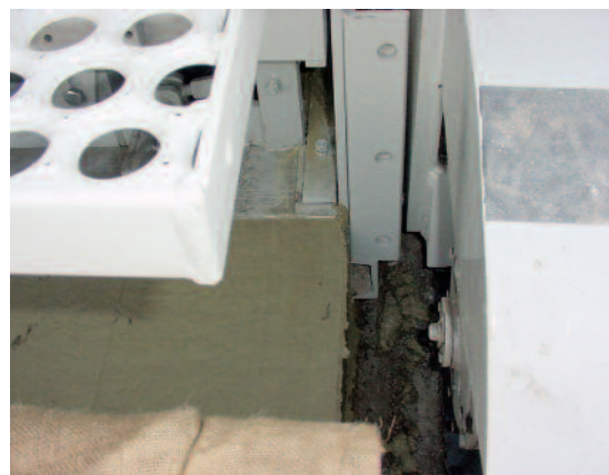
The side-forms are connected to the tracks.
