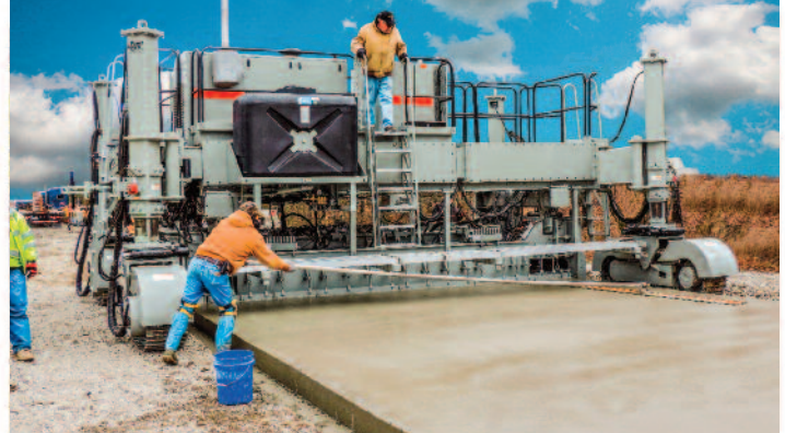
▲ Power Pavers Full-Sized, 4-Track SF-2404 Slip-Form Paver
