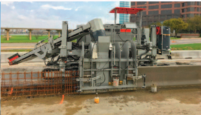
▲ Power Curbers 7700 Multipurpose Slip-Form Machine Pouring Barrier
