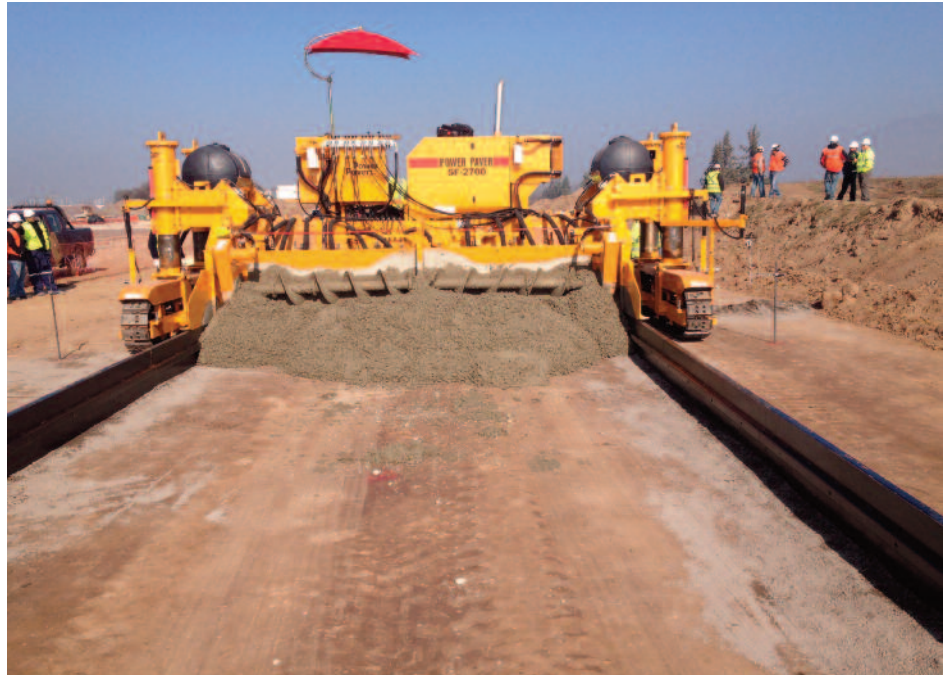
The SF-1700 and SF-2700 frames can be extended to pour over fixed forms.
