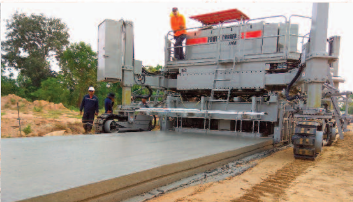
▲ Power Curbers 7700 Multipurpose Slip-Form Machine Paving
