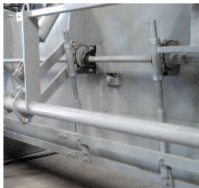
Tamper bar and vibrator mount/lift.
