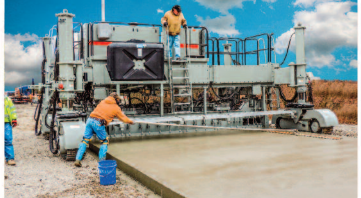
▲ Power Pavers Full-Sized, 4-Track SF-2404 Slip-Form Paver
