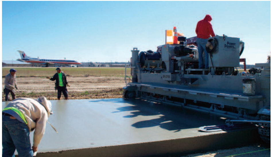
SF-2700 paving an airport.
