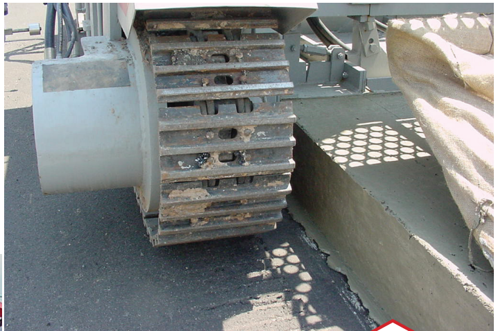
Paving a thin layer of white topping over asphalt.
