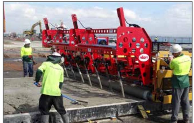
For over twenty five years, Allen has been the preferred source for triple roller tube pavers. These unique form riding machines can do the work of larger more expensive pavers in many applications. Triple roller tube pavers are easy to transport and setup as they have lighter weights than traditional slip-form pavers. These pavers are great for confined, urban job sites where forms are going to be used or concrete streets, parking lots, shoulders, ramps, approaches, airfields and more.
